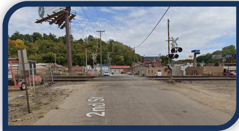
Figure 48 – 2 nd Street Crossing
