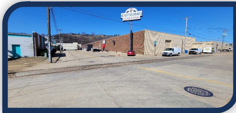
Figure 12 - Salina Street Crossing
